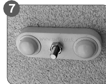
7 Insert plug, fixing and screw cap.
