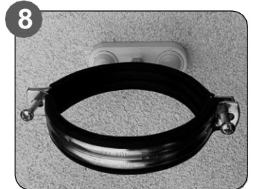
8 Secure the pipe clamp.
