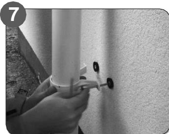
7 Attach neoprene washer and insert tube into system.
