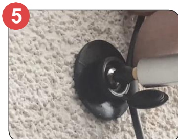
5 Insert screw utilising the screw cap fix item required (shown - p-clip attaching cable).
