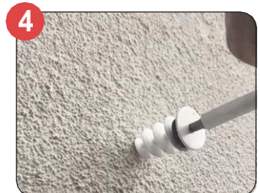
4 Carefully Screw into render using a T30 torx head screw driver. Note: Using mechanical means may burr the fitting.
