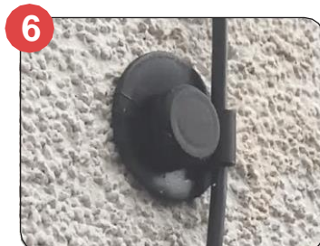
6 Job complete and water tight.
